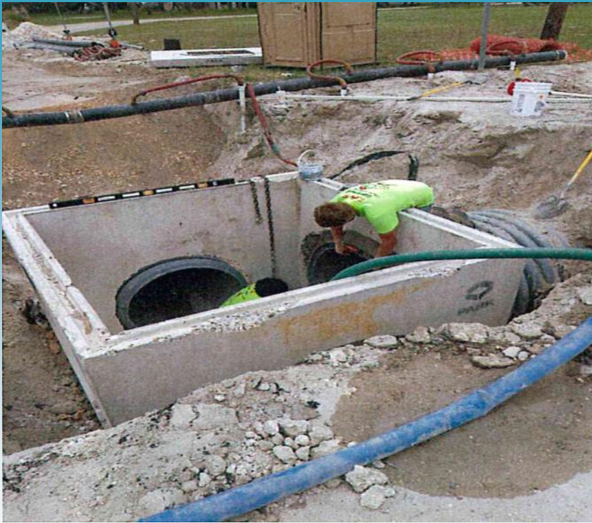
Contractor JJ Fox employees working on the Highland Stormwater project
